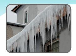
cicles form when **the roof surface temperature** rises above **0** °**C** or when **snow** melts on a roof due to **sunshine**. The melted water drops down and when reaching a **colder** area at the eaves, **freezes** and forms gradually growing icicles. Icicles may **cause trauma** to pedestrians or **damage to vehicles** when they fall down; their weight may **break power lines** and sometimes even the constructions of buildings and facilities.
